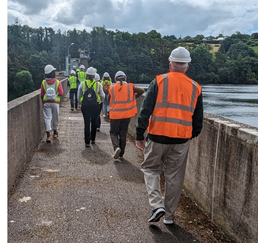
"The highlight of the trip was a day where we explored the River Lee," said civil engineering student Alysha Jarvis. "We started by stopping at Inniscarra Dam and learning about how the dam was built, along with trekking to the top to see the engineering of the gates that control the water flow."
