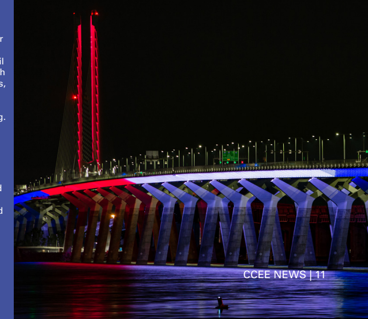
The Samuel De Champlain Bridge illuminates the water below at night. Photo courtesy of Infrastructure Canada.
