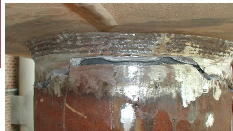
Pictured above are undesirable weld fractures and retrofit scheme.
