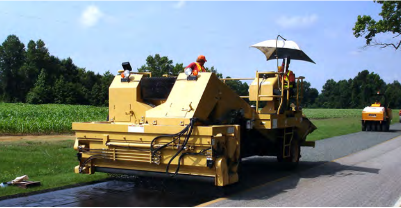
Construction of preservation surface treatment to extend service life of pavement
