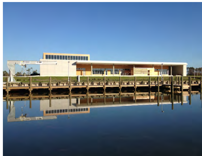
The Institute's Marine Services Building
