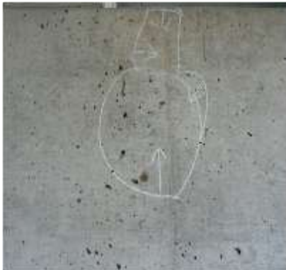
Photo and IRT image of a concrete pier cap that is a candidate for repair using GFRP (WVDOH)
