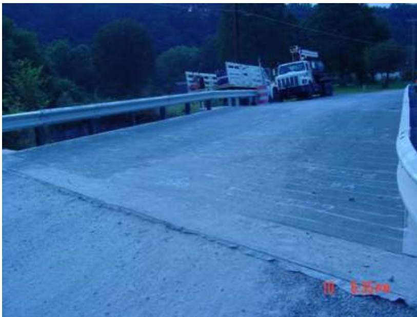
La Chein FRP Bridge, Monroe County, WV
